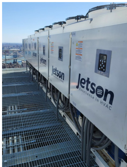
Array Installation (Modular)
